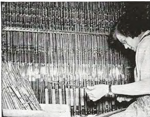
Montague makes rods for every kind of fishing known to man, be it fresh-water or salt. Here the windings and guides of fly rods are given careful coats of preservative just before final varnishing.
