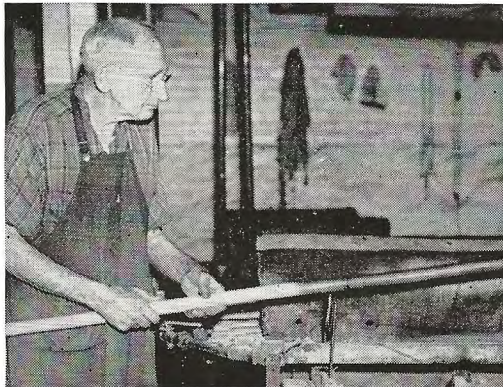
Flame-finishing a Montague Rod. This process tempers the cane, gives it a rich color and—most important—the added life and resiliency for which Montagues are famous.
